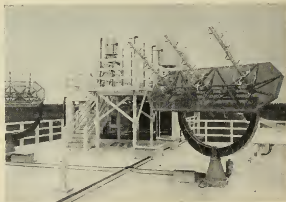
WIDE VARIETY of receiving antennas atop the FCA center monitors, locates any troublesome radio or radar signals.
