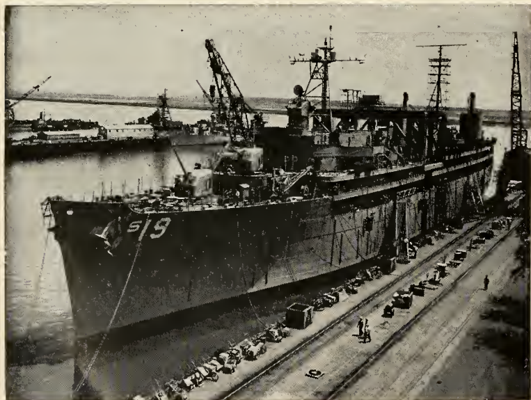
SUBMARINE REPAIR tender Proteus undergoes completion at Charleston Naval Base. The massive bridge crane above deck amidships will be used to handle 28,000-lb. Polaris IRBM's and a 120-ton nuclear waste container.
