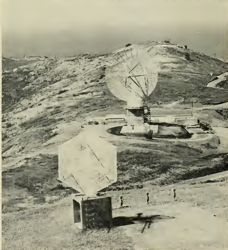
SIGNALS SENT from Kaena Point, Hawaii can change orbital period on Discoverer satellites. Tracking station is one of six used in program.
