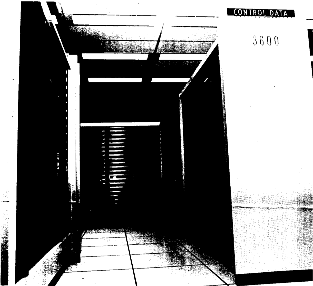
COMPUTER ELEMENTS —Elements of the Control Data 3600 computer are shown in the MSC Data Reduction Complex in Building 12.
