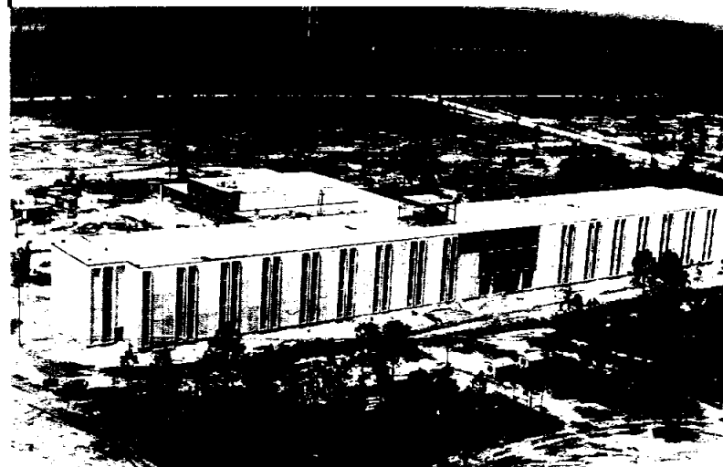
MTO FACILITY —The main Laboratory and Engineering Building at the NASA-Marshall Space Flight Center's Mississippi Test Operations, nearing completion, will serve as administrative headquarters for NASA and its contractors. The Laboratory and Engineering Building is one of about 30 major construction projects underway at a cost of some $250 million. At present, facilities are under construction for static testing the first two stages of the Saturn V moon rocket. Operations are expected to begin in late 1965.
