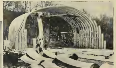
Panels are heavy-gauge steel—double-curved and corrugated for rugged strength. Bolt together—self-supporting.
