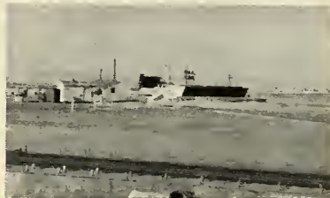
SUNKEN OBSERVATION blockhouse dominates rocket acceleration track's end. Booster storage is in background.
