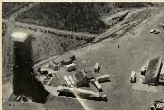
A SHROUDED Atlas missile arrives at Convair's Sycamore Canyon facility for captive testing. Part of the two-level reinforced concrete blockhouse, which serves as a test control station, can be seen at upper right. Liquid oxygen propellant for the missile is stored in a tank behind bunker.
