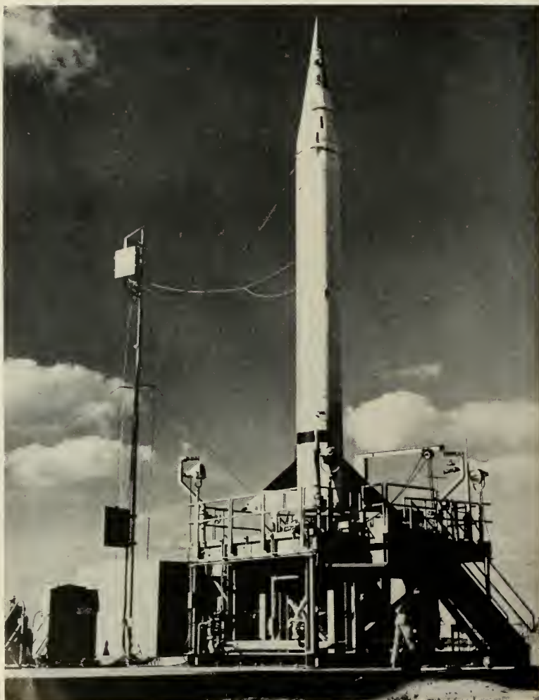
This exclusive shot of the VANGUARD launching platform shows Navy VIKING ready to go. Loewy-Hydropress Div. of Baldwin-Lima-Hamilton Corp. designed and built the structure.
