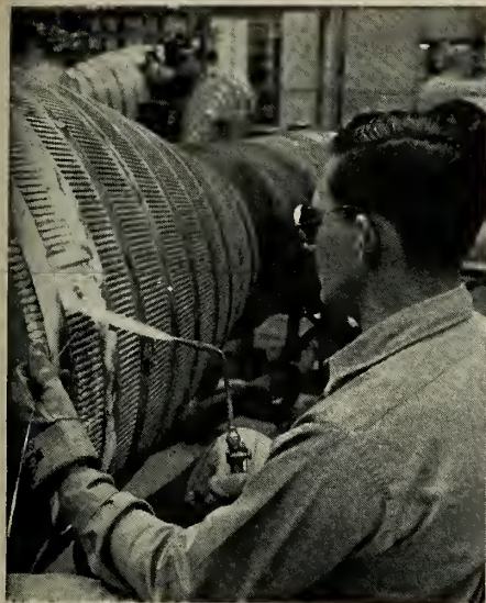
MOST CRUCIAL operation is tube soldering.
