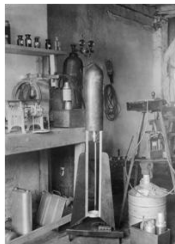
Fig.6 New Version of HW1 with fins
