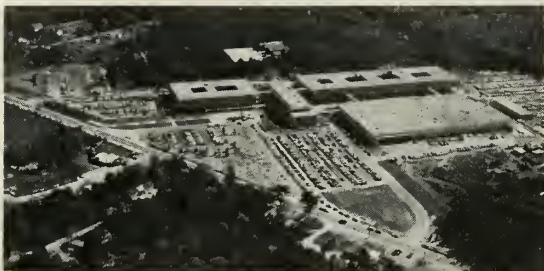
$23 MILLION research center ready.
