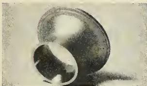
Tungsten cup being drawn preliminary to shaping into missile hardware.
