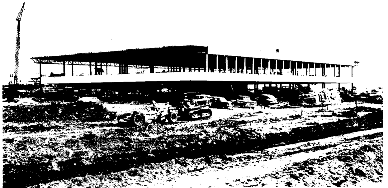
CENTRAL DATA Office Building at Clear Lake is taking on shape and character with the installation of the exterior wall panels. Scheduled for completion in early September of this year, the two-story facility will provide office space for the Technical Information and Computation and Data Reduction Divisions, together with computer rooms and data storage.
