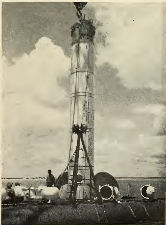
LAUNCHING TUBE for R&D Polaris missiles is one of two on the stern of the Test Ship Observation Island . This one can be tipped at a variety of angles.
