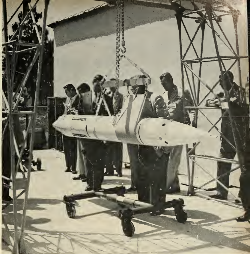
HOISTING SLING used with portable A-frame and adjustable missile storage stand provides flexible, mobile handling gear for storage, assembly, maintenance.
