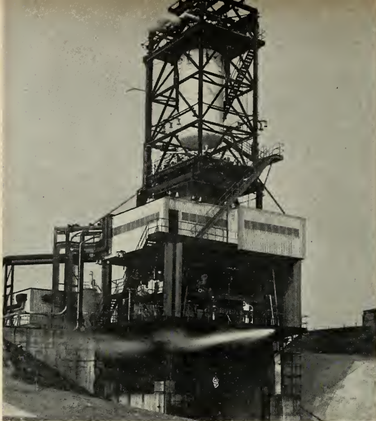
ABOVE: Close-up of a Rocket Engine Test Stand.
