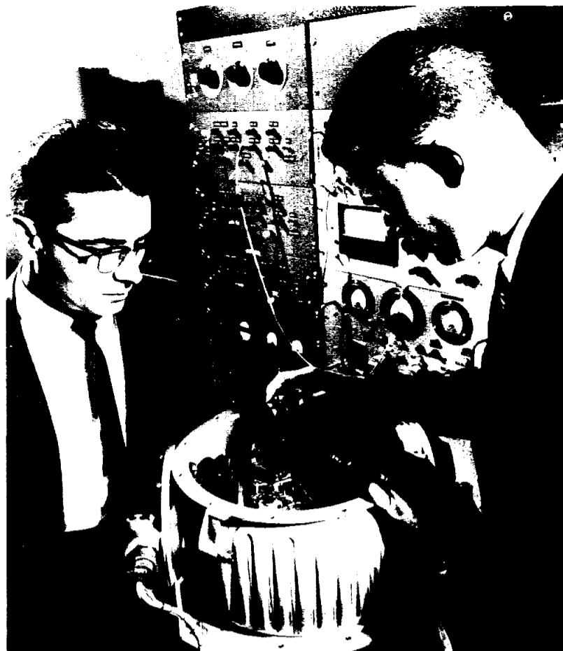
MOON GUIDANCE —An acceleration-sensing space speedometer is mounted in a test model of the ball-shaped inertial navigation system "platform" that will help guide U. S. astronauts to the moon and back. These units being manufactured by the Sperry Gyroscope Company under contract to NASA for the Apollo project, will sense changes in speed and direction of a vehicle.
