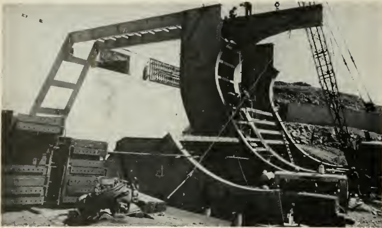
Soon to be completed, this test stand at the Denver plant of Martin will be used for early static testing of the TITAN.
