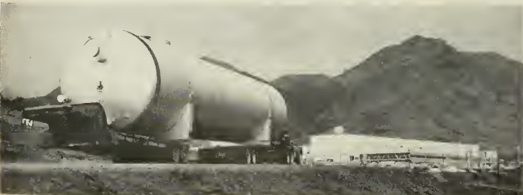
This is a 28,000-gallon, stainless steel "thermos bottle" type tank which will be used for liquid oxygen and other fuels. The tank is 11 feet 6 inches in diameter, and 75 feet in length.
