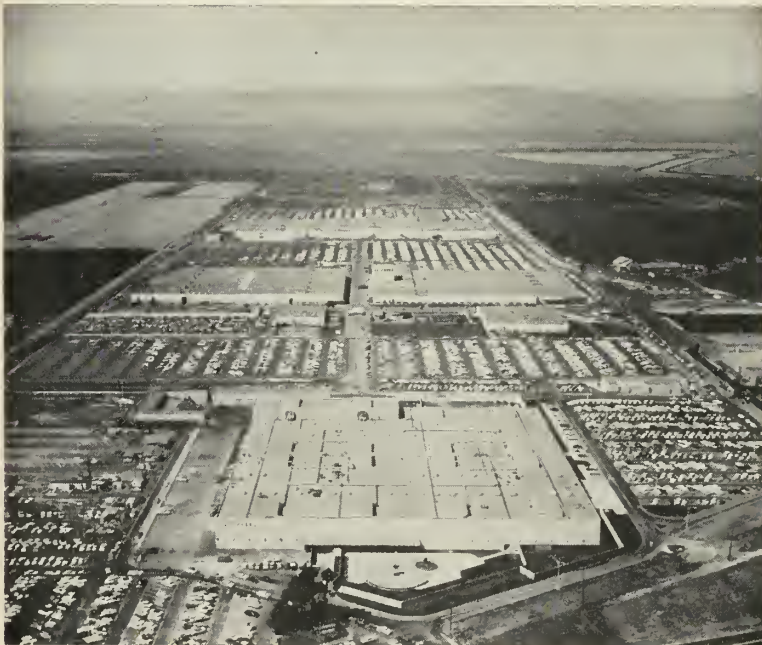
SPRAWLING OVER 645 acres, Lockheed Missiles and Space Division's Sunnyvale site includes recently activated headquarters for Discoverer , Midas and Samos projects.
