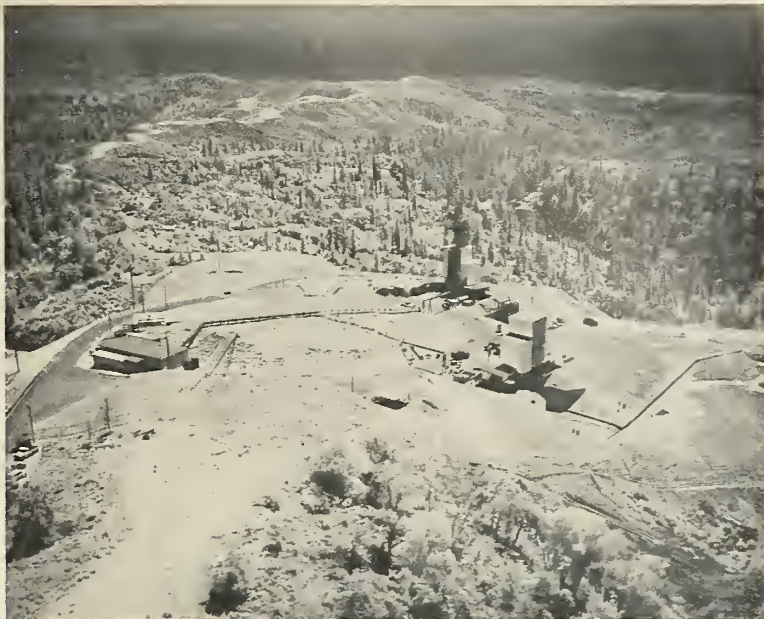
TWO TEST stands tower over LMSD's Santa Cruz site, with the Pacific Ocean in the background. The site covers 4000 acres and has a payroll of some 484 persons.
