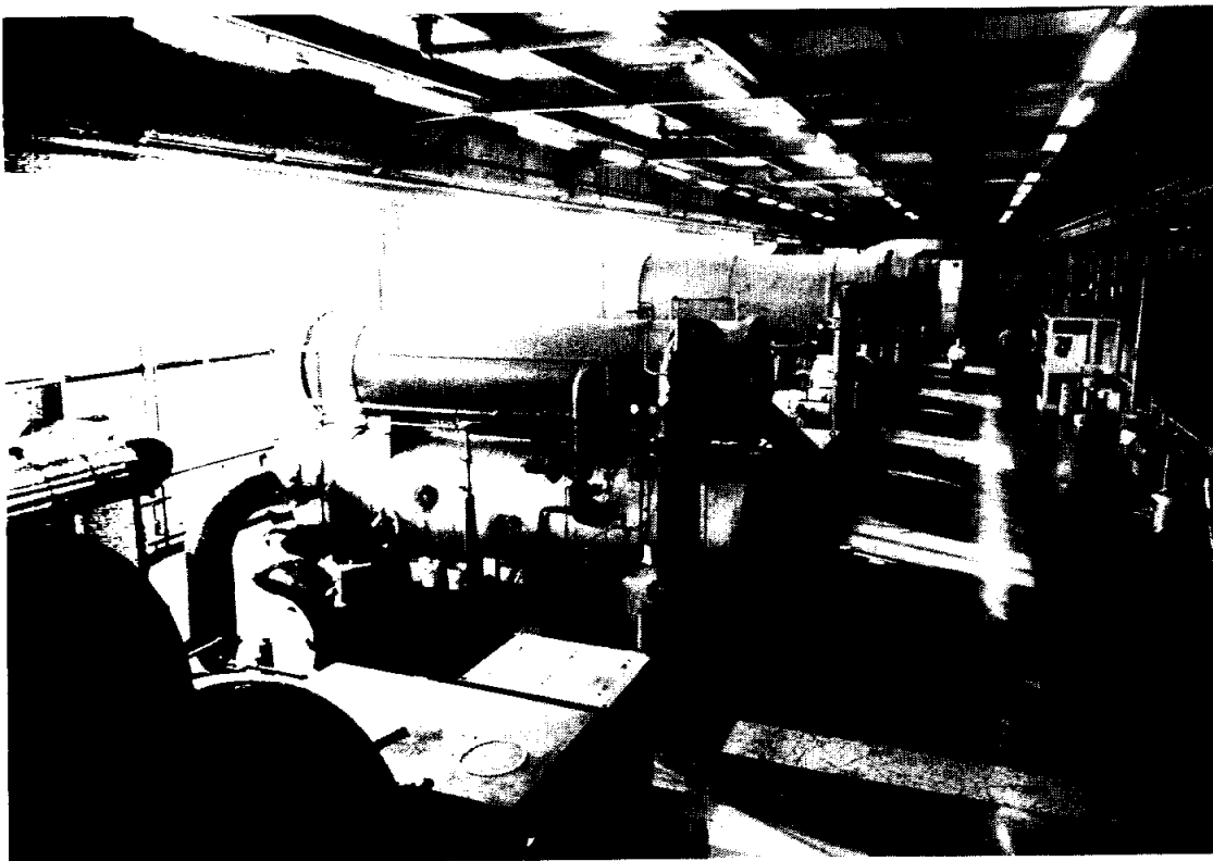
Above: L.K. Fuller, a Pan Am supervisor in the Central Heating and Cooling Plant, and Don Sims, a utility operator, stand among the Bldg. 24 chillers that—holiday or no holiday—keep JSC buildings cool. Many buildings need to be cooled even during the winter because of the heat radiated by computers. Right: Electrician Larry Miller, a Pan Am World Services utility operator, works on a circuit breaker in Bldg. 24.
