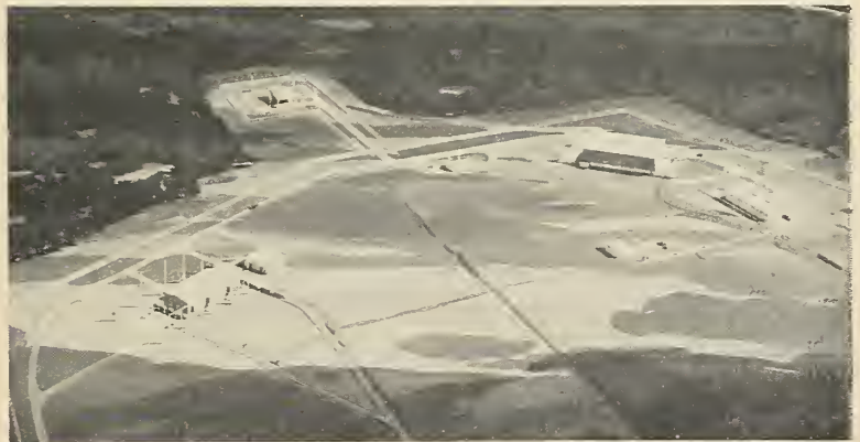
LAYOUT OF Polaris Depot, the Navy's new operational missile assembly facility near Charleston, S.C., is shown in an architect's drawing. The buildings lying in the semicircle from left to right are: Missile Assembly Building, Equipment Building, Motor Processing Building, Re-entry Body Building, Container Building, Inert Processing Building. Not shown are the widely spaced rows of magazines where warheads and motors will be stored.
