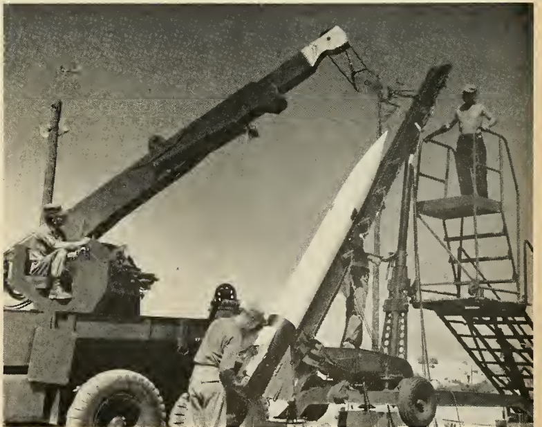
EVEN THE SIMPLE free-flight Little John requires an array of ground support gear. Army
