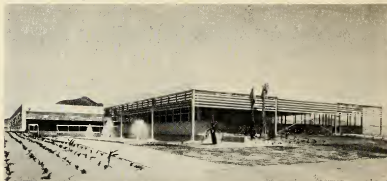
PACKARD BELL ELECTRONICS $750,000 plant covers 53,000 sq. ft. of proposed 350,000-sq.-ft. electronics complex at Newbury Park, Conejo Valley, Calif. Its Technical Products Div., advanced electronics equipment manufacturers, will be housed here.
