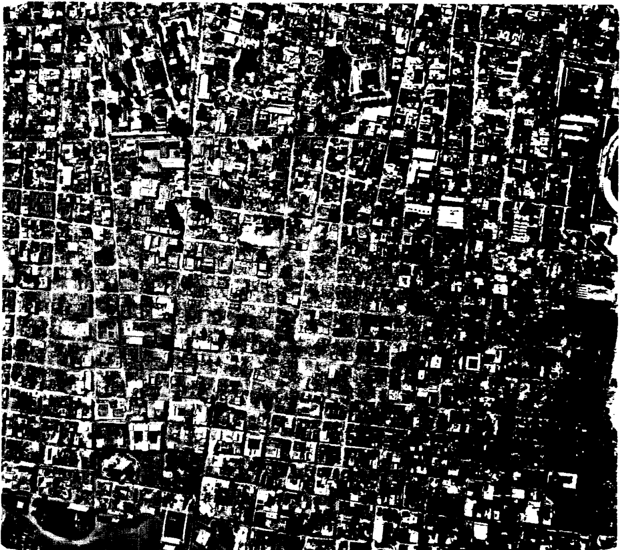
NICARAGUAN EARTHQUAKE DAMAGE—A low-altitude aerial view of the Central American city of Managua, Nicaragua, showing extensive damage caused by the earthquake of December 23, 1972. This photograph of the capital city was taken at an altitude of 3,000 feet six days after the disastrous earthquake. This picture was taken from a NASA C-130 earth observations aircraft, using Kodak Ektachrome (serial) film. Some buildings and rubble are still burning.
