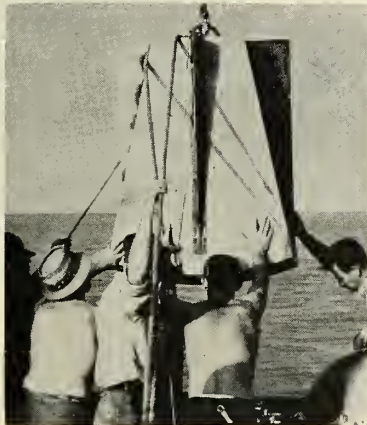
FIRST OVERBOARD is anchor, cut loose by explosive bolts before AIDA ascends.
