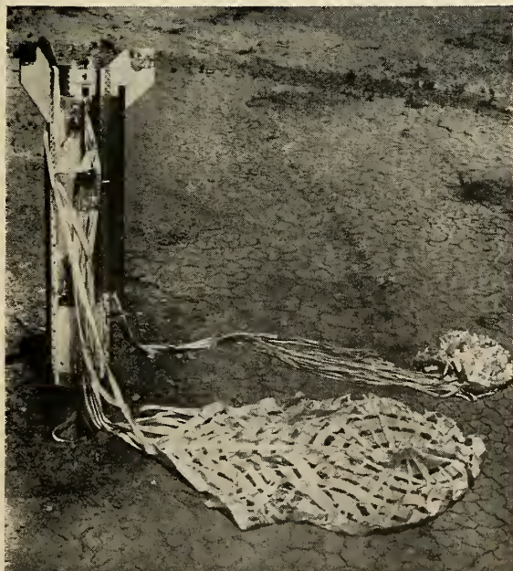
CREE RESEARCH missile is shown just after successful soft impact. The recovery chute is still attached.
