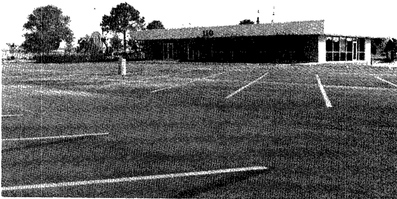
Construction of the new Bldg. 110 is complete inside and out, and security personnel will begin moving into the new badging building on Thursday.
