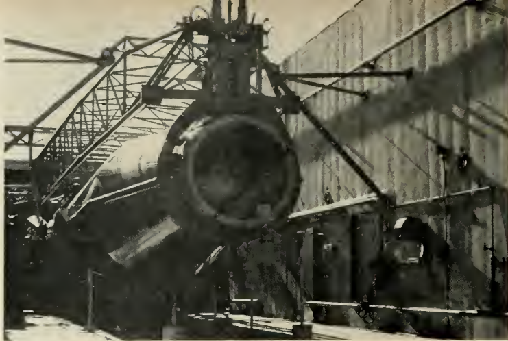
ATLAS and erector system in "coffin" type, aboveground site. Roof is opened. Vandenberg has three such installations. The erector system is almost identical to standard Atlas transporter-erector. This and other illustrations are first photos, taken exclusively by M/R.
