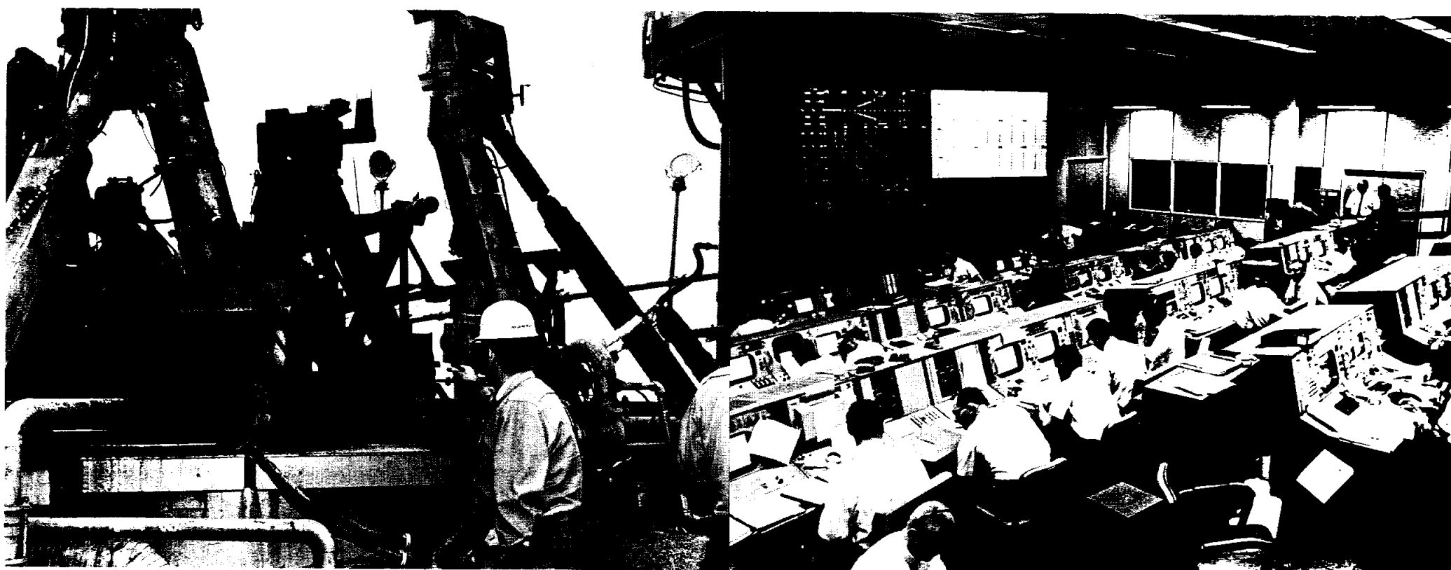
SCORCH CHECK —Damage to Launch Complex 19 from the Gemini VII launch was minimal, and the Gemini VI launch vehicle was erected atop the same structure early the following morning.
