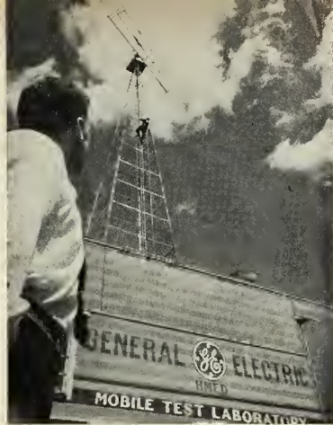
THIS 100-ft. antenna at General Electric's Heavy Military Electronics Department, Syracuse, N.Y., was used to receive signals during recent field tests of the Phantom broad-band communication system.
