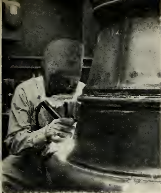
HELIARC welding the exterior of a double-walled thrust chamber for Rocketdyne's Redstone engine.
