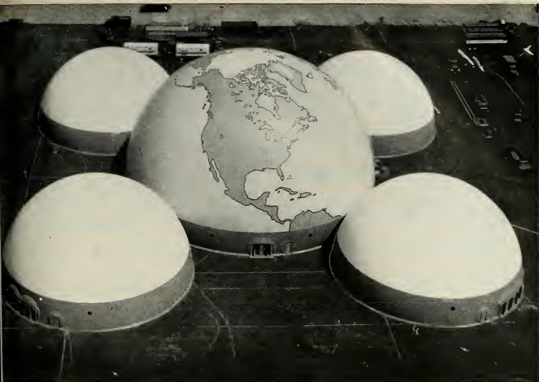
The Pentadome structure, developed by an industrial team in cooperation with the U. S. Army Quartermaster Corps, was designed to meet Ordnance Corps requirements for a missile maintenance shelter.
