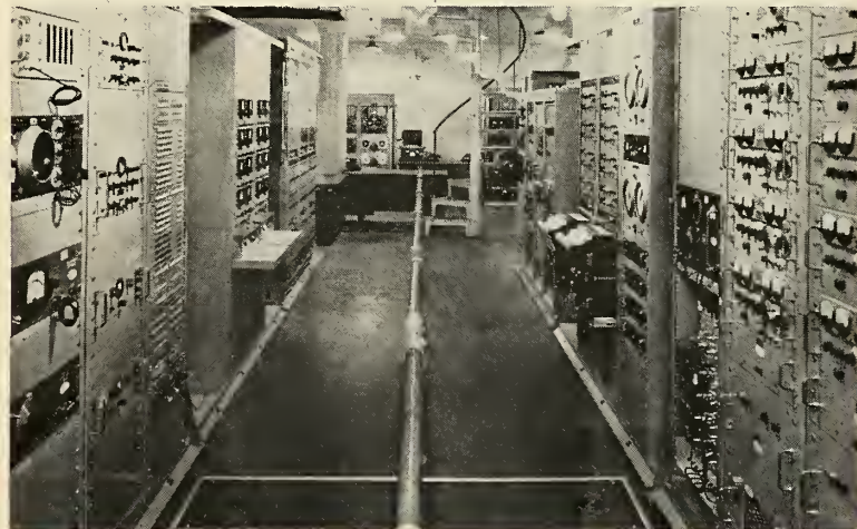
TELEMETRY receiving station installed aboard picket ships of the Pacific Missile Range which are deployed to supplement range stations on various Pacific islands.
