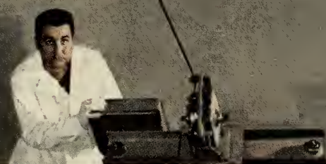
Ultra high strength wire ribbon being formed into a rocket case on specially designed wrapping machine.
