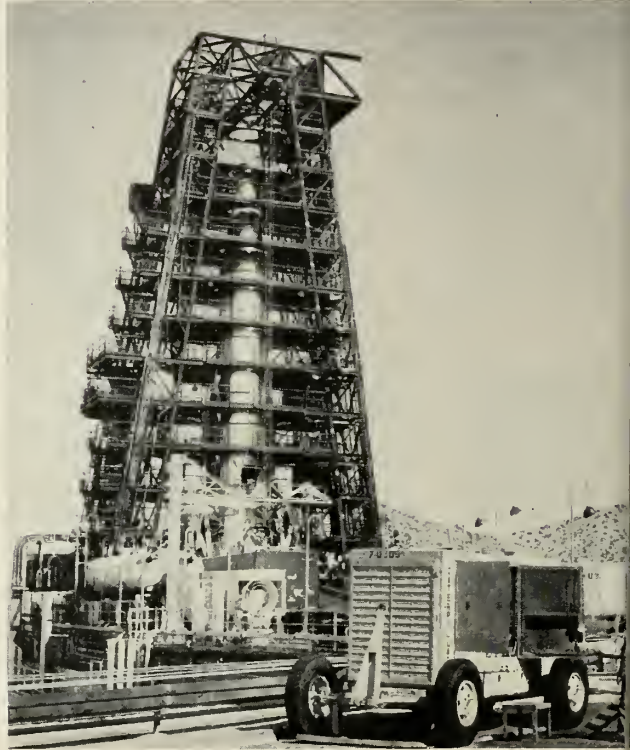
At Edwards Air Force Base in California, power for testing the precision electronic control circuits of the Atlas missile is supplied by two Cat D375 Diesel Electric Sets. They meet the triple requirement of portability, dependability and accurate control.
