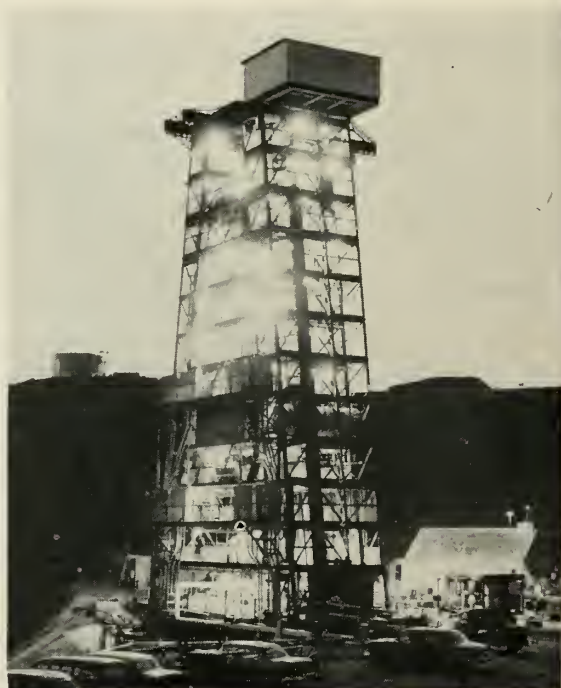
STATIONARY Atlas engine testing stand was Kaiser's first. They collaborated with Convair on its research and design. Convair controlled support in Atlas program.
