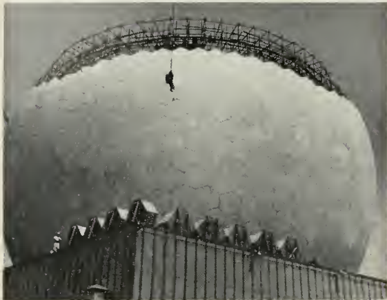
FIG. 3 (at left)—Recently completed near New Jersey Turnpike just east of the Camden-Philadelphia area, is a prototype of similar installations to be constructed in the Far North. The dome will provide protection for huge antennas inside. It was fabricated by Goodyear Aircraft. FIG. 4 (at right)—Artist's cutaway drawing shows in-location installation at a Far Northern site of BMEWS tracking antenna and supporting pedestal being fabricated by Goodyear under a multimillion-dollar RCA contract.
