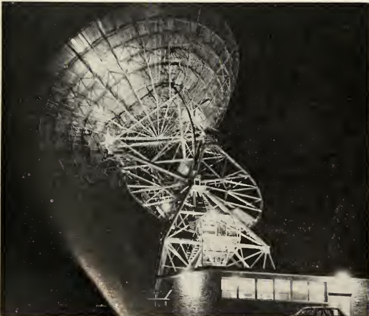
SEARCHING FOR extra-terrestrial life, 85-foot diameter radio telescope listens for artificial signals emanating from stars 11 light years from earth.
