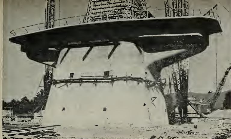
INCREASED SEARCH range will come from 140-ft.-diameter radio telescope whose foundation is shown rising from a field in Green Bank, W.Va.
