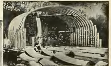
Panels are heavy-gauge steel — double-curved and corrugated for rugged strength. Bolt together — self-supporting.
