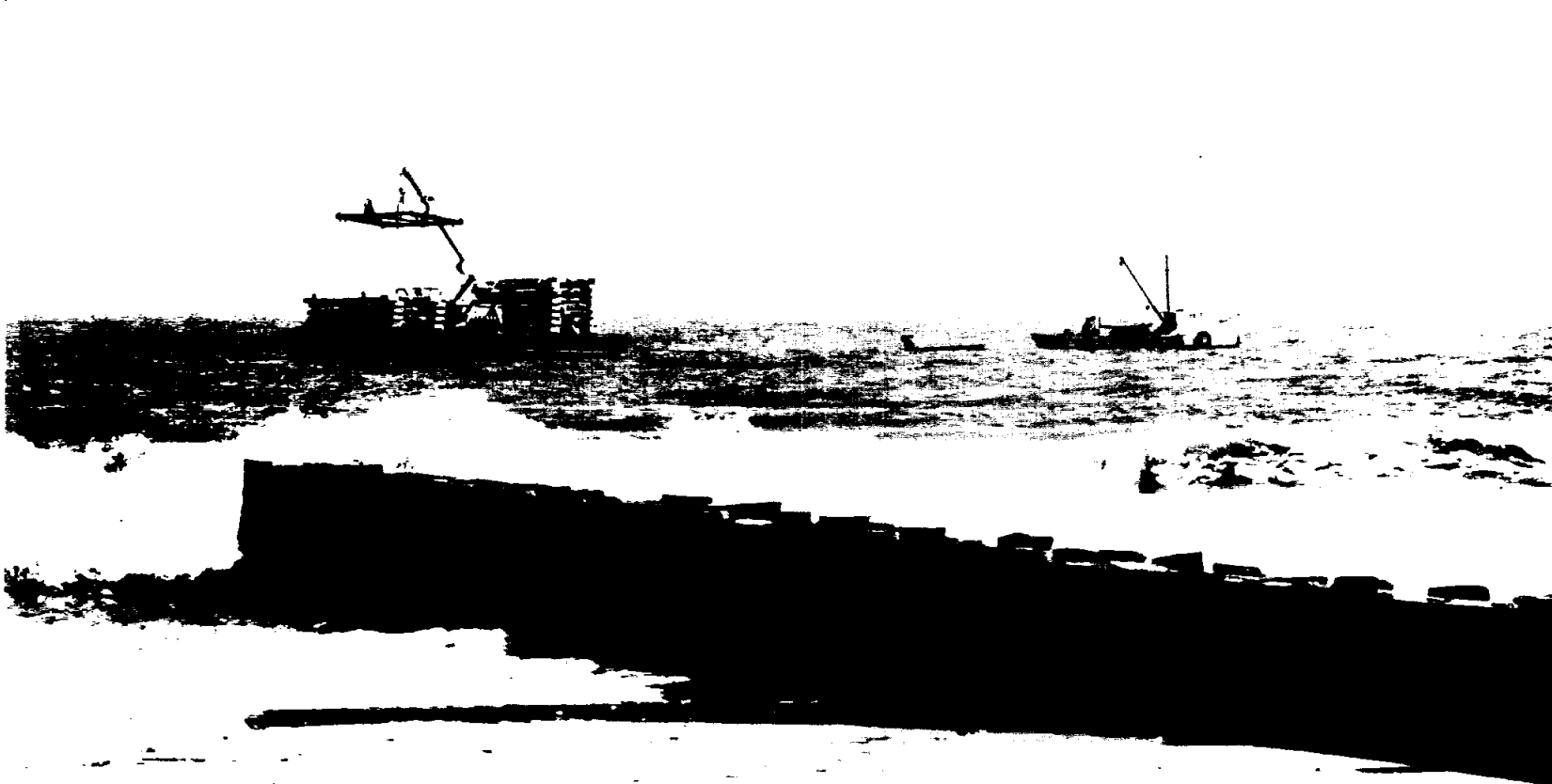
ERSATZ SEAWEED—Metal frames with artificial plastic seaweed attached are lowered from a barge offshore of the NASA Wallops Station, Va., as part of an experiment to develop means of retarding sea erosion. The fake seaweed fronds float underwater like the real thing and attract barnacles, water blisters and sea ferns as well as inducing sand particles in suspension to drop to the bottom. The reefs also attract fish where there were none earlier.
