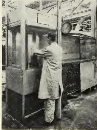
METAL POWDERS , ceramics and cermets are compacted in hooded 270-ton vertical hydraulic presses in R&D laboratory.
