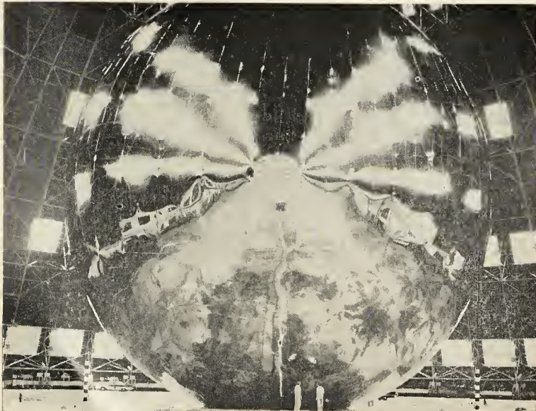
ECHO SATELLITE is shown during ground inflation tests. Forty thousand lbs. of air is required to inflate the sphere on the ground, only a few lbs. in orbit.
