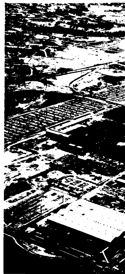
AMERICA'S LARGEST ROCKET PLANT —Sacramento, Calif., dedicated to the res- America's military and space programs. sible for all phases of Gemini engine development, manufacturing and support.
