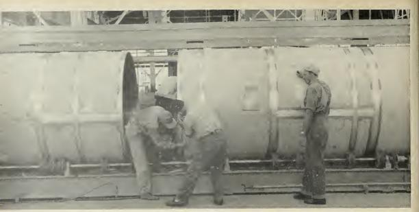
Fig. 3-Workmen welding sections of the JUPITER-C. New techniques have contributed many diverse uses of both old and new metals.
