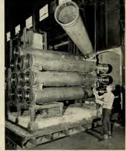
In an assembly fixture, the three principal parts of the motor—nozzle, tube, and forward ring—are welded into a single unit (Above).
