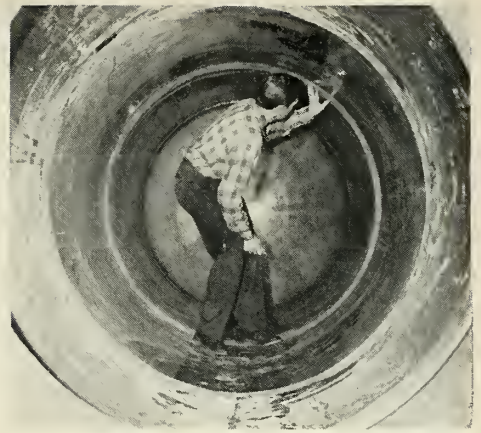
SIXTY-INCH diameter tube demonstrates fabrication size possible with epoxy laminations.
