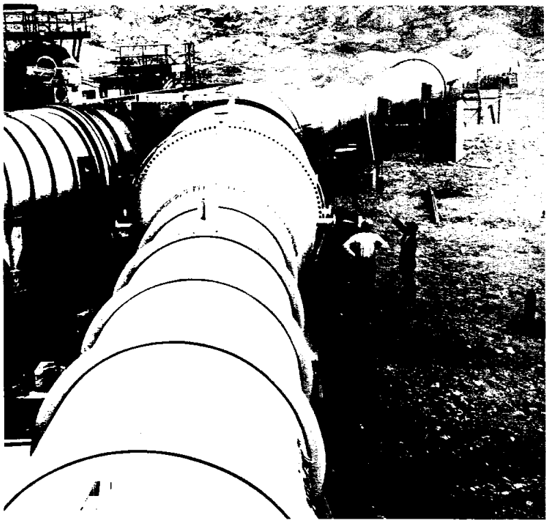
ALTITUDE TEST FACILITY —Lunar Excursion Module (LEM) engine being developed by Rocketdyne, a division of North American Aviation, Inc. is ground tested in this facility at Nevada Field Laboratory. One of largest vacuum test structures in U.S., facility is capable of simulating pressures encountered at altitude of 150,000 ft. Facility stretches 260 feet across high plateau overlooking Nevada desert.
