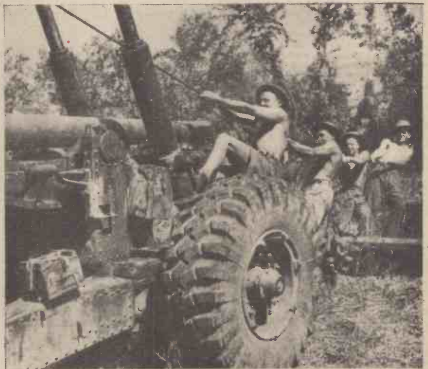
In the Far Eastern theatre of war a famous Artillery Regiment carried out repairs to their medium guns on the field. The illustration shows a gun crew hauling a gun barrel into position.
