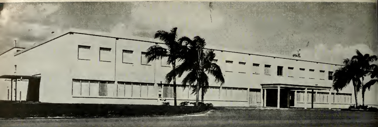
MINNEAPOLIS-HONEYWELL'S gyroscope and inertial guidance facility—surrounded by a moat to minimize vibration.
