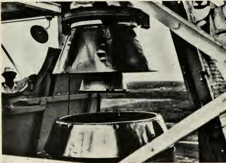
SECOND STAGE comes into position for joining with Primary Stage of Thor.
