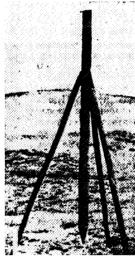
FIGURE 150. Rocket pile driver
