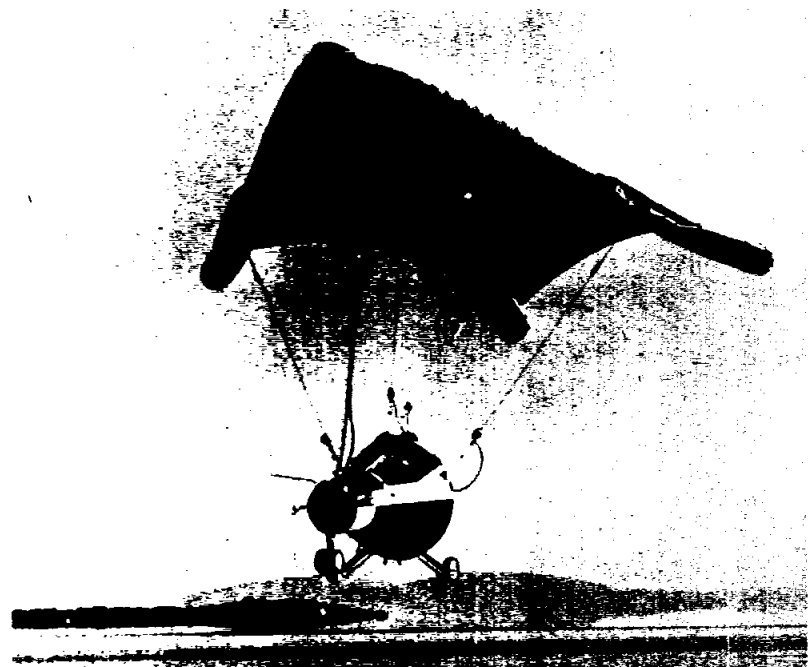
PARAGLIDER SUCCESS—Last Wednesday the paraglider was towed aloft by a helicopter and then it glided back to earth while still attached to the copter by a cable. Pilot E. P. Hetzel rides to earth in the spacecraft suspended from the paraglider at Edwards AFB. A successful deployment test was also completed with an unmanned vehicle.
