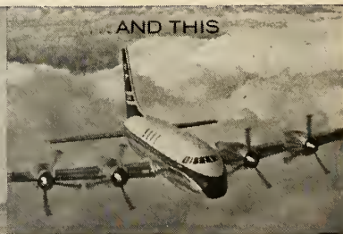
The Bristol Siddeley Proteus powers the Britannia airliner.
