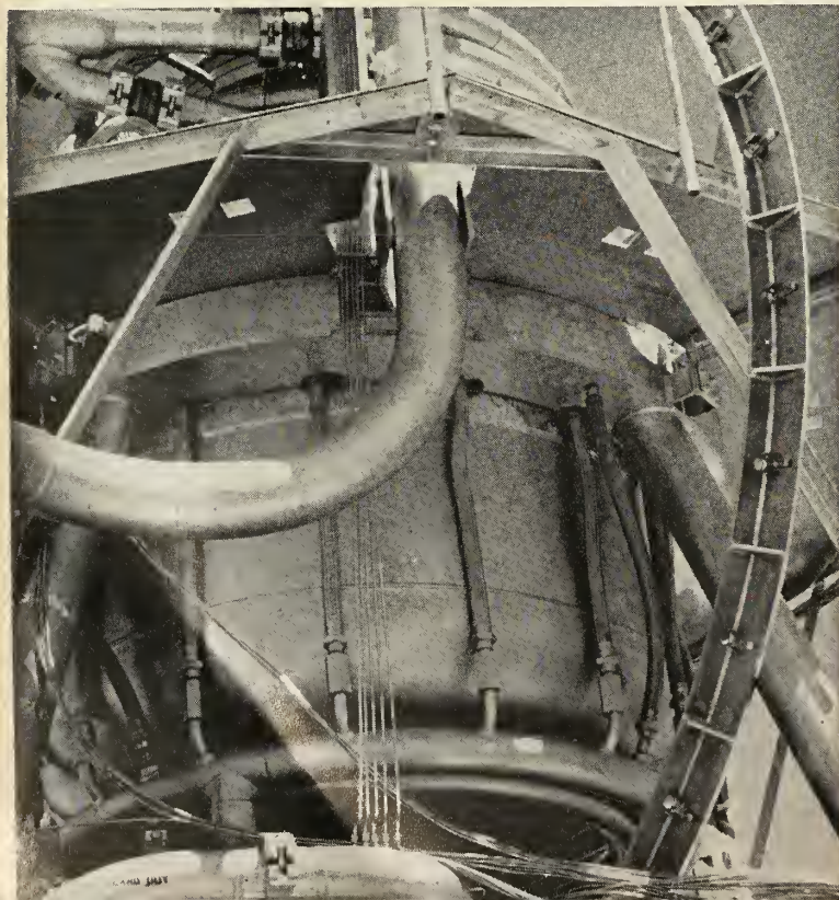
BELOW: Close-up of Kiwi-A-Prime reactor cold flow unit shows ducting of system used for handling liquids, instrumentation wiring and structural member arrangement.
