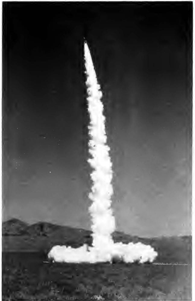
Fig. 6. This 10-ft.-long "GAPA" (Ground to Air Pilotless Aircraft), made by Boeing, is a potential defence against high altitude enemy aircraft.
