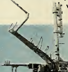
1956-NAVAHO G26 Transporter-Erector, Launch Pedestal, Flame Deflector, Service Stands and Tower
