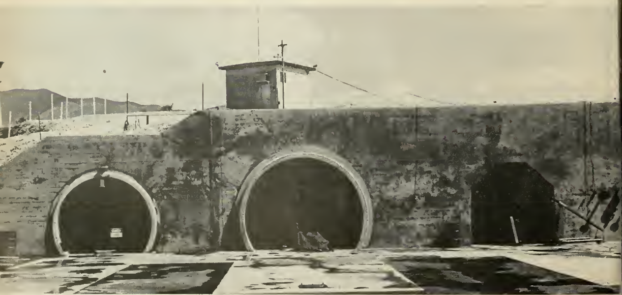
Latest addition to Grand Central's facilities—three test bays for static firing small and medium-sized solid-propellant rocket motors.
