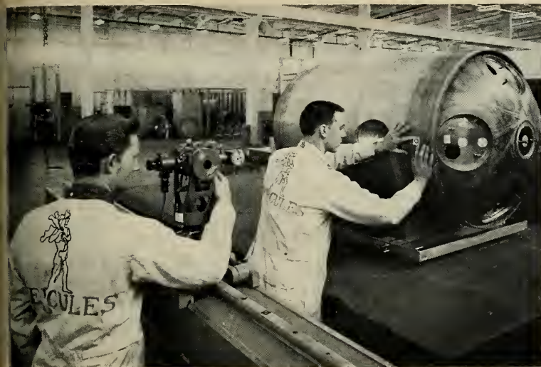
OPTICAL CHECK OF nozzle port alignment is made on third stage's Spiralloy case. Ports can be integrally wound into case with accuracy within 3 minutes of angle.
